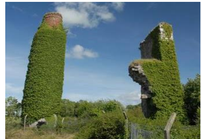
The old Kilbricken Mine, a Victorian era Pb-Zn mine worked 1834-1854. A Cornish Engine House is still visible today.
