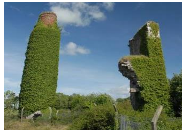
The old Kilbricken Mine, a Victorian era Pb-Zn mine worked 1834-1854. A Cornish Engine House is still visible today.
